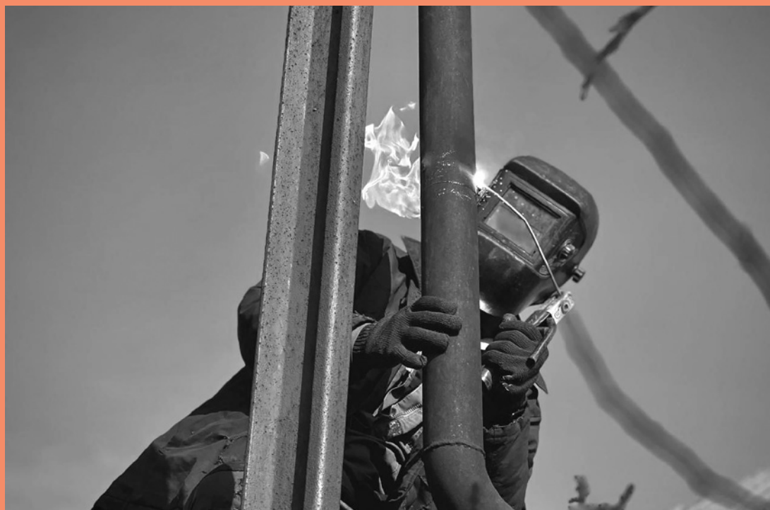
Replacement of gas pipes Photo: Angelina Fesenko
